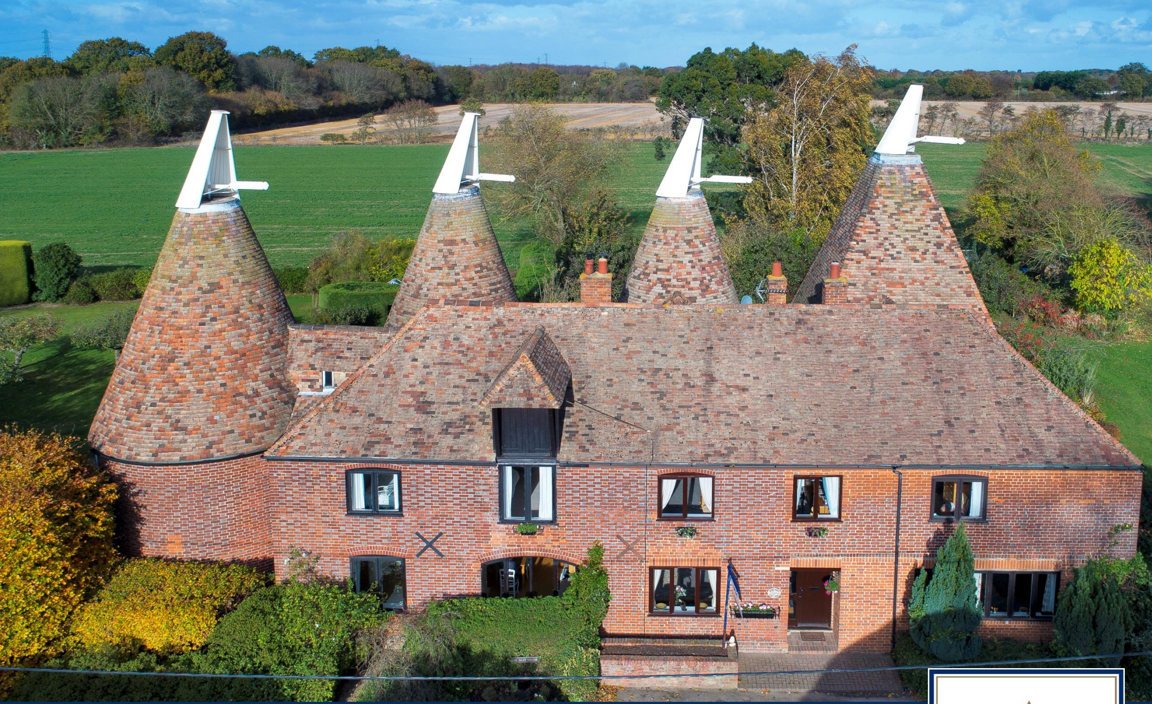
Hode Lane, Bridge, Canterbury
